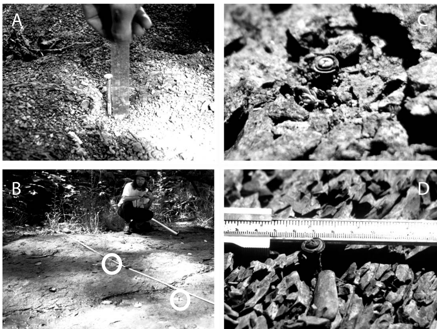
Figure 7. One to several years of bedrock lowering indicated by erosion pins in (A) W.F. Satsop, (B) Black Creek, (C) Walker Creek (site 1), and (D) S.F. Eel. See Table 2 for details. Note that pin protrusion above the surface indicates pervasive lowering, not localized scour or damage from installation. Lowering in the Satsop and Eel is by detachment of centimeter-sized weathered fragments during high flow. Lowering at Black and Walker Creeks is by folia generation and removal during high flow.
